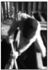
Nick Testa works on house flooring
